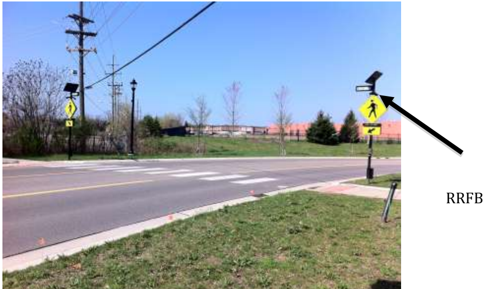
Figure 1. Condition B: RRFB on Grand River Avenue
