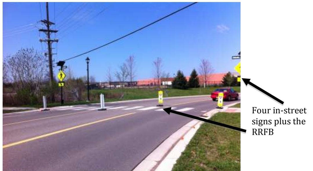
Figure 5. Condition F: RRFB Plus Gateway Treatment
