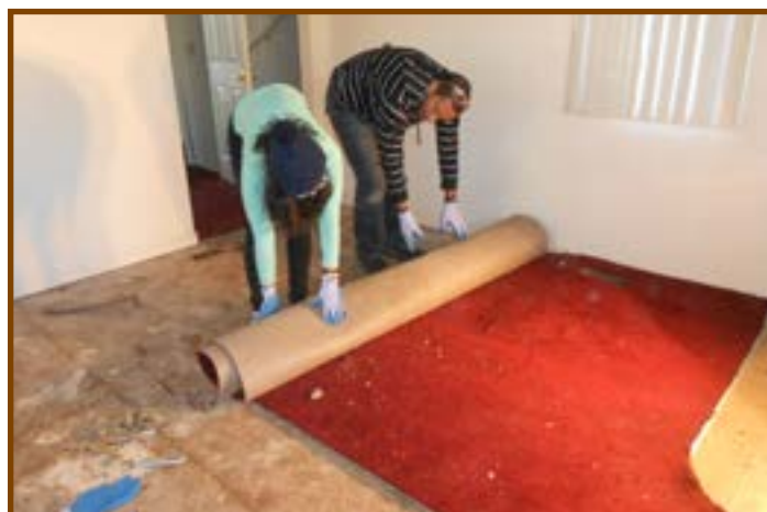
WMU students helping on a Kalamazoo Habitat for Humanity project
