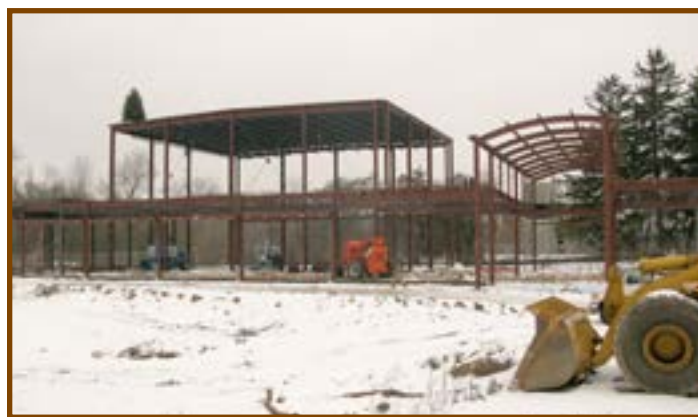
Zhang Legacy Collections Center construction showing the "topping out" tree
