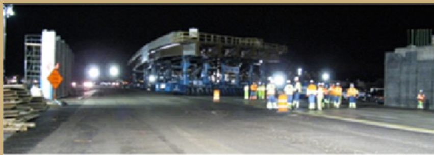
Above and Below: Bridge being moved to its final location
