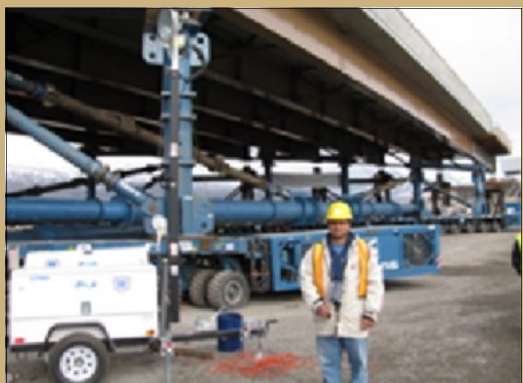
Above: Bridge supported by 4 SPMTs
