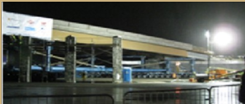
Above and Below: Bridge being moved to its final location
