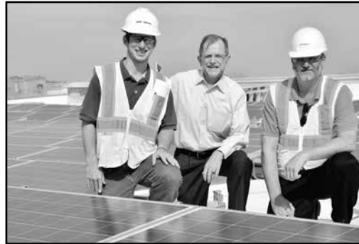
Dunn, center, and two Miller-Davis reps check out Sangren Hall's new solar panels. (Photo by Mike Lanka)
