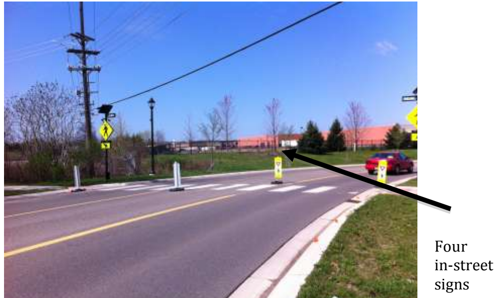
Figure 4. Condition E: Gateway Treatment
