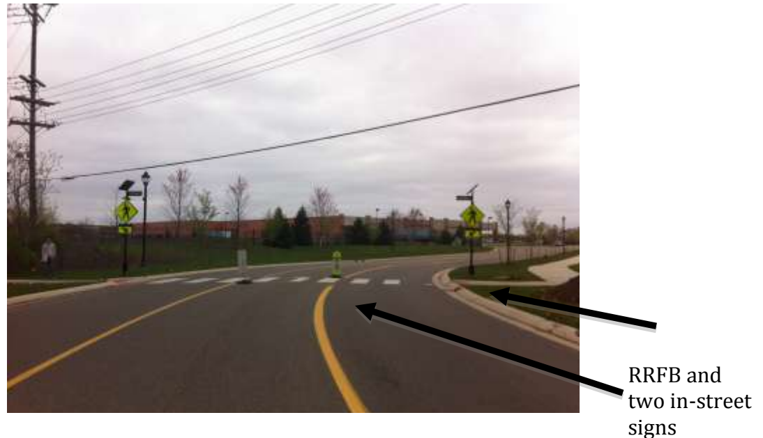
Figure 3. Condition D: RRFB and Two In-street Signs
