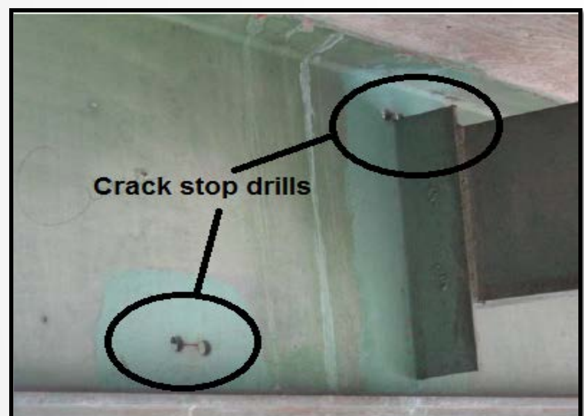
Figure 3. Retrofitting fatigue cracks (Source: Zhao et al. 2013)
