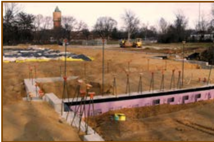
WMU Legacy Collections Center: Foundations laid and Cement curing
