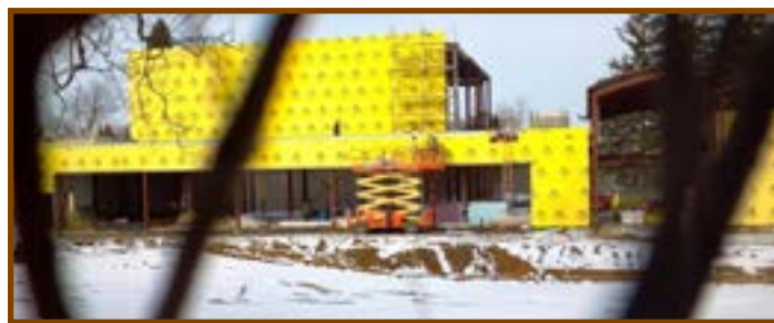
Zhang Legacy Collections Center takes shape during February
