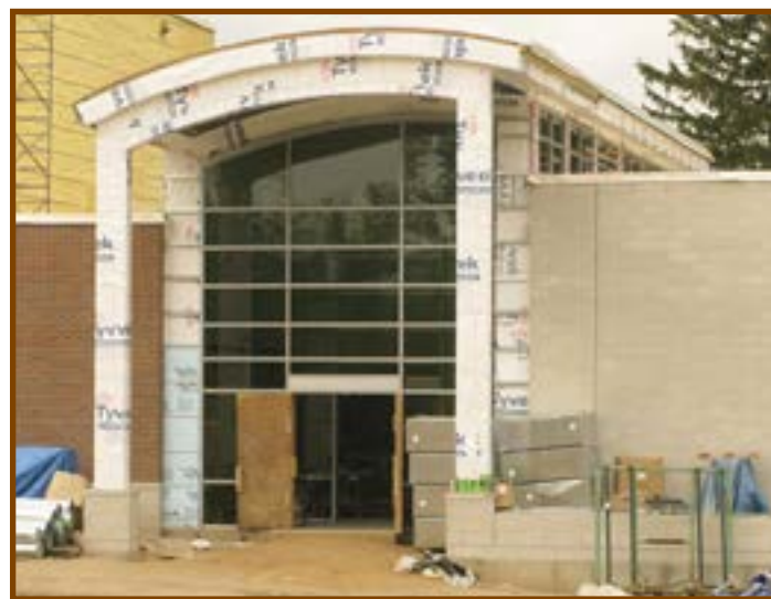
Front window-wall is newly installed
