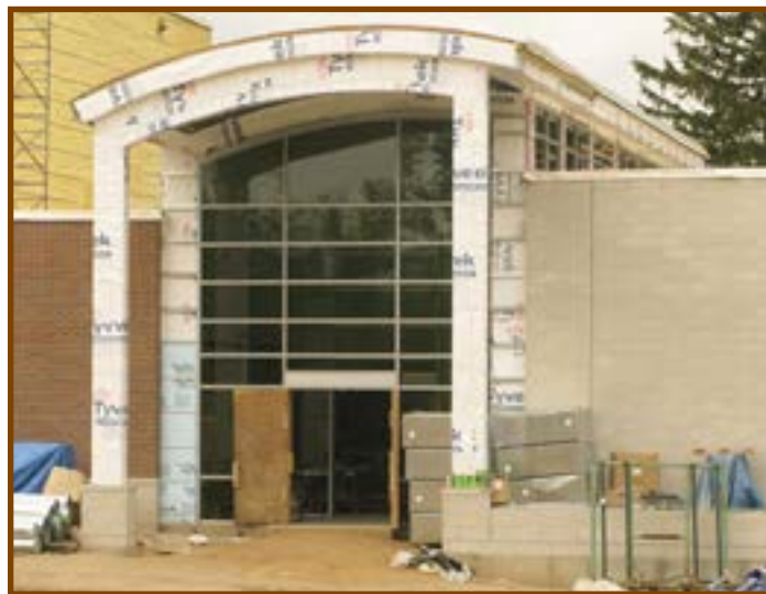
Front window-wall is newly installed
