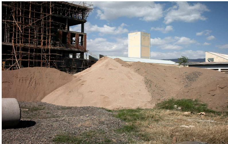
**Plate 4** Storage and variation of sand quality in a typical construction site.
