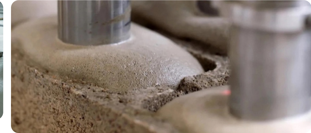
Figure 62. Holcim Cast-in-place Concrete
