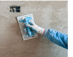
Figure 95. Hempcrete Plastering
