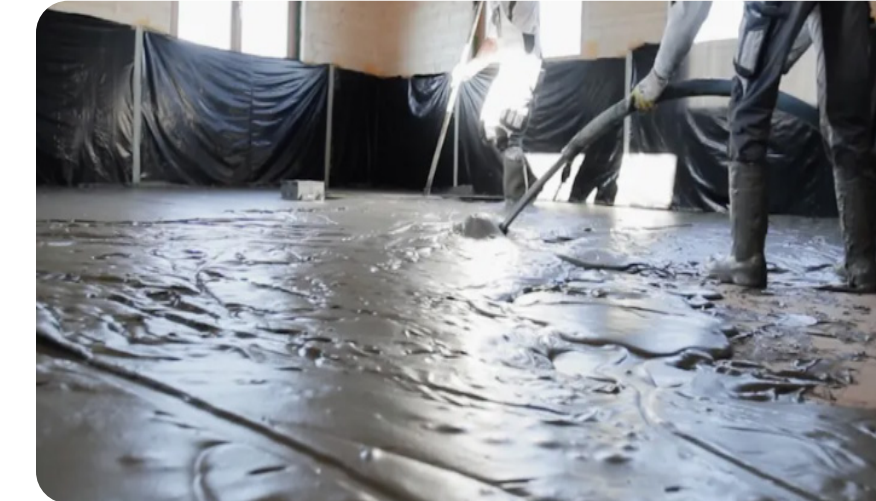
Figure 60. Holcim Poured Concrete
