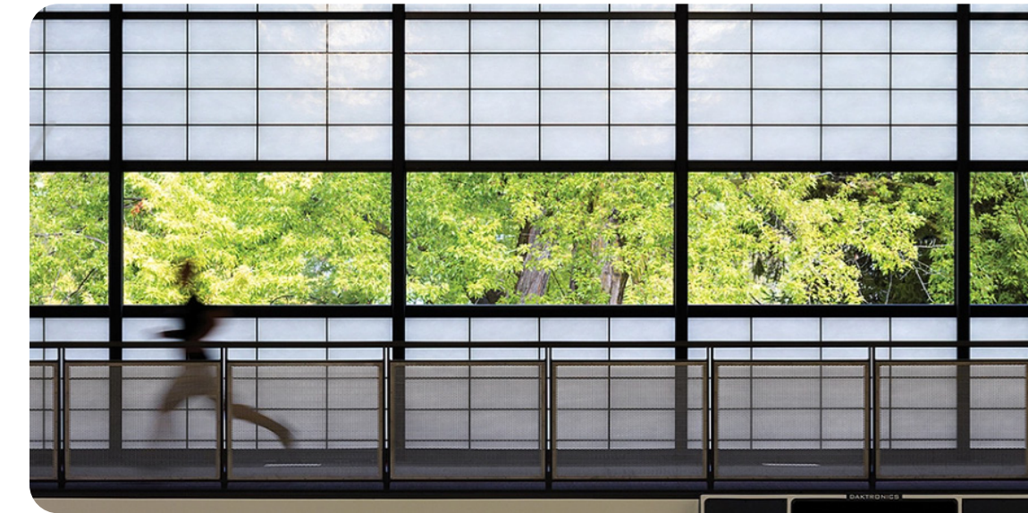
Figure 52. Kalwall Facade System Example
