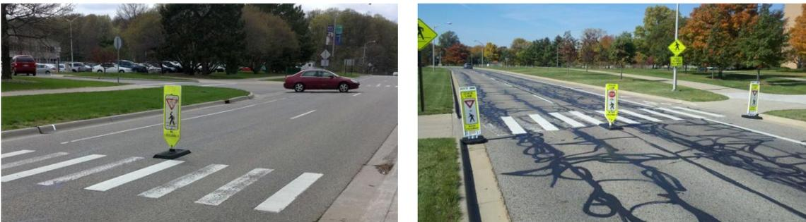
Figure 1. Gateway with gutter pan.
