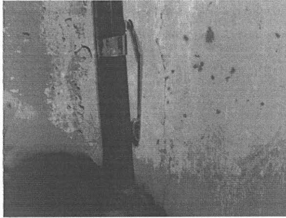
(b) Deck Bottom Surface Cracking
