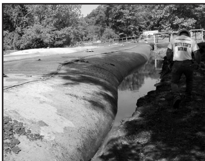
Left photo: Large filter bags have removed decades of fine materials from the Goldsworth Valley Pond. Right photo: An electrician wires fixtures that will light up Heritage Hall's new West Overlook. (Photos by Jeanne Baron)
