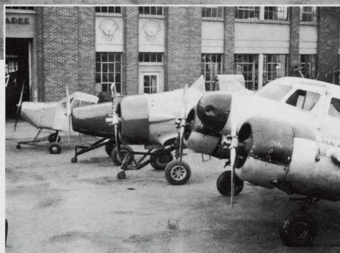
Run-up and trouble-shooting engine stands, c.1950 (outside Mechanical Trades Building). Left to right: Aeronca TG-5, Fairchild PT-19, North American AT-6, and Cessna AT-17. Western acquired several engines and trainers as military surplus following WWII. The engines and cockpits were mounted on moveable stands. After students would work on the engines, they were wheeled out to the parking lot and fired up. The roar of the engines was a common sound in the 1950s and early 1960s. The twin engine Cessna at the right presented a particular challenge, as it was 18 feet wide and the doorway to the Mechanical Trades Building was 16 feet. Herb Ellinger rigged the stand with a special pivoting wheel from the landing gear of another aircraft and with a little "chopping" to the wings and frame was able to maneuver the engine stand through the doorway. Note the carved cement aircraft engines in the Mechanical Trades Building (erected 1941).
