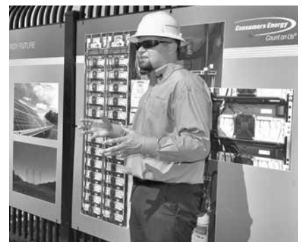
With the aid of a banner at the event, Consumers Energy Project Manager Nathan Washburn explains how the new facility and its racks of batteries work. (Photo by Mike Lanka)
