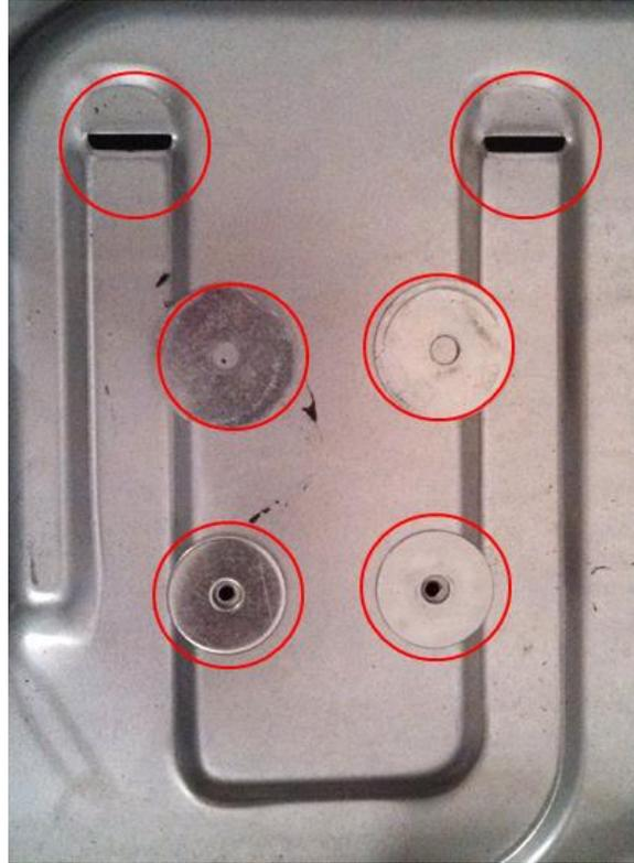
Figure 48: Secondary bracket redesign, incorporating washers.
