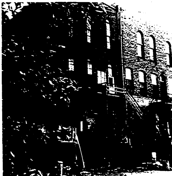
In the rear the buildings are four stories.
