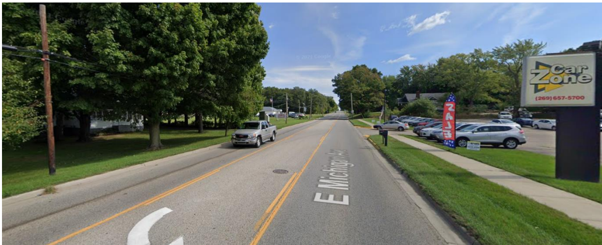
Figure H.10 shows the end of the public water line in Paw Paw. The hydrant on the left side of the image marks the end water line.
