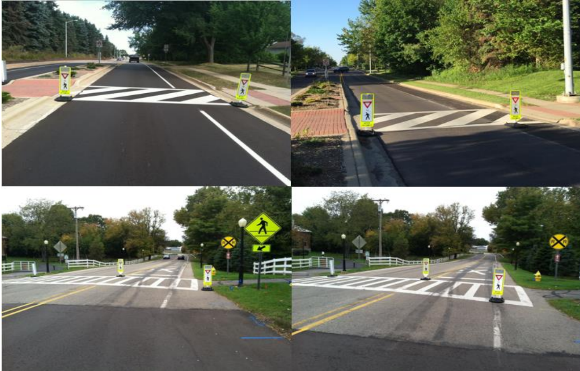
Figure 3. Oakland Drive trail crossing wide (top left) and narrow (top right) configurations; Garden Avenue trail crossing wide (middle left) and narrow (middle right) configurations.
