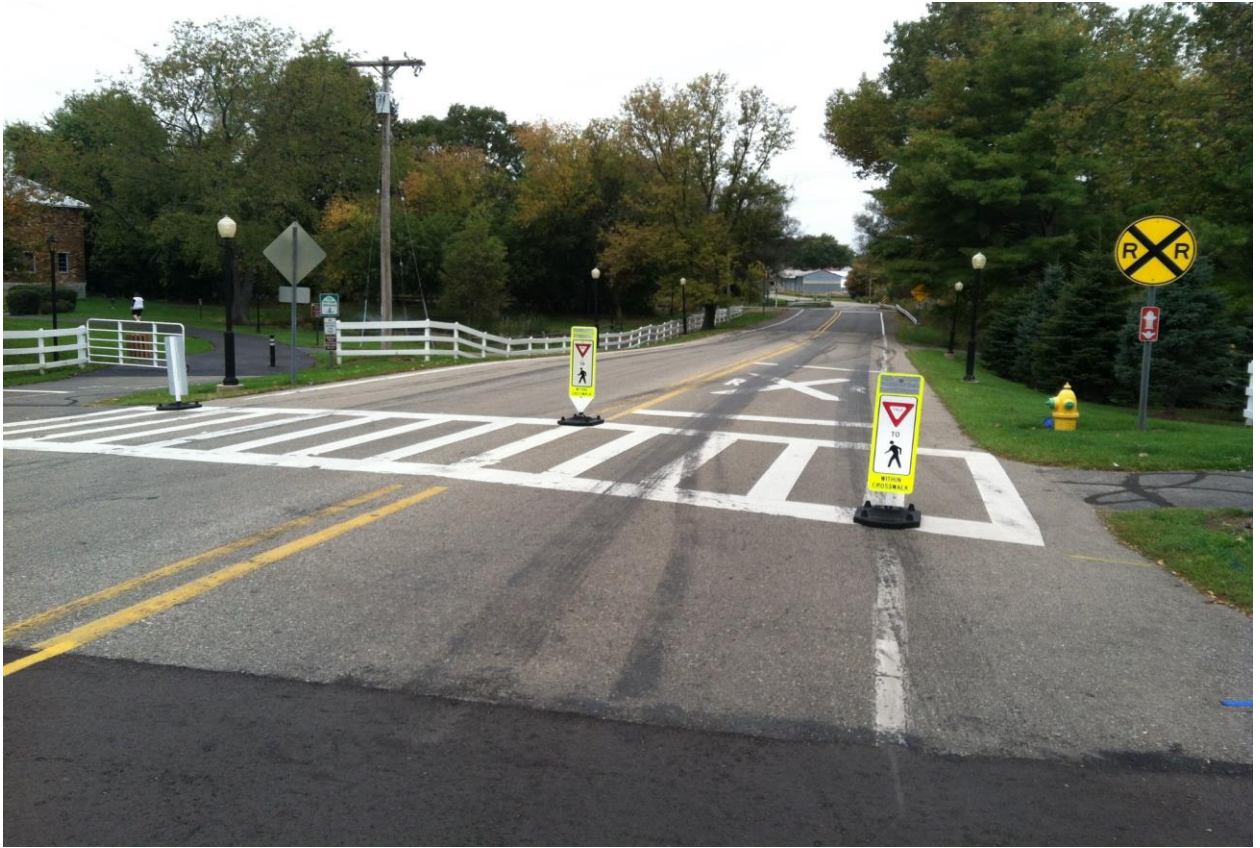
Figure 2. Garden Lane location, facing East.
