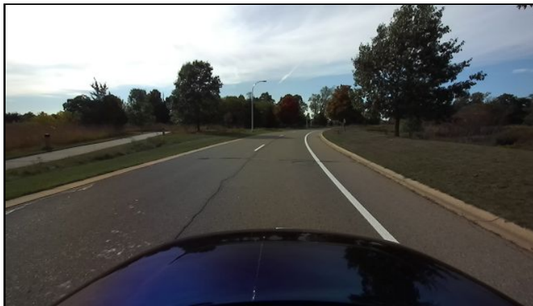
Figure 18. Frame from image data collected over the Campus Drive loop.
